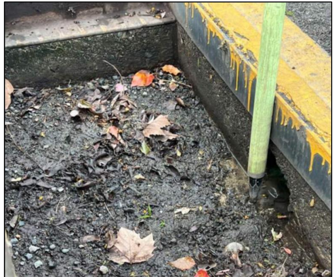
Figure 13 - Existing Area Drain
