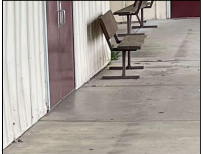
Figure 12 - Existing Door Conditions
