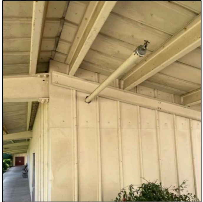
Figure 14 - Existing Water Line
