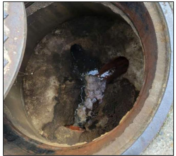
Figure 16 - Existing Manhole Outlet
